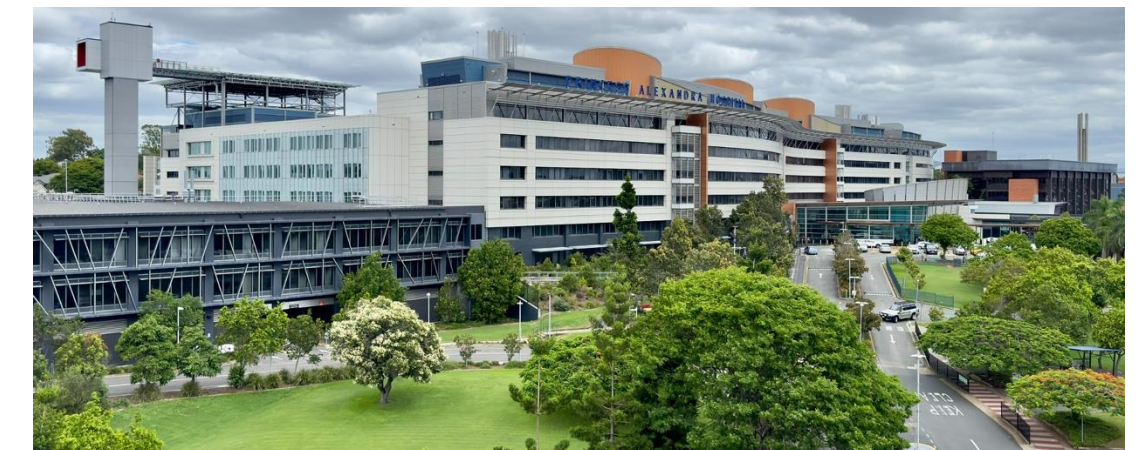
Queensland Government Metro South Health
